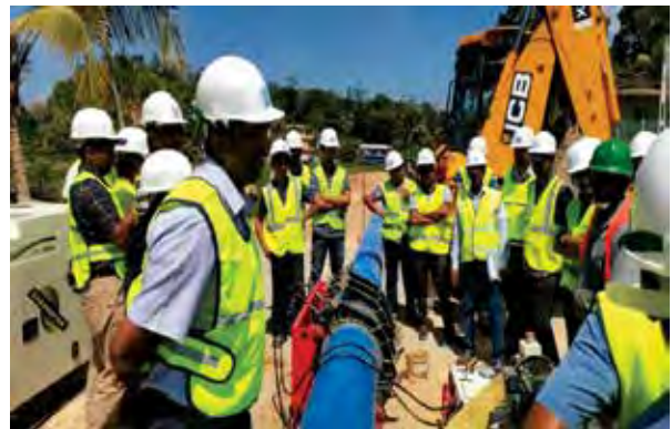
Field Visit on Stage IV Water Supply Project – Matara
